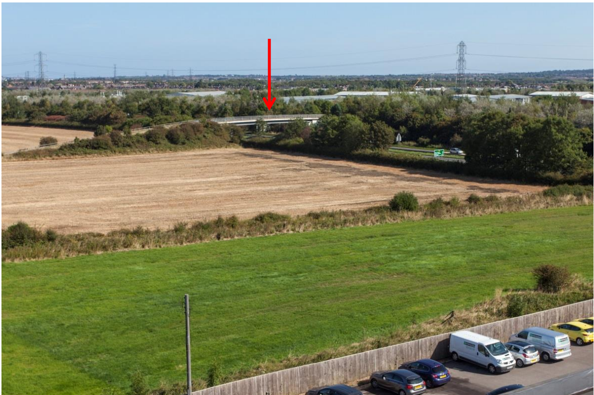
Plate 3-1: Bridleway B28 - accommodation bridge over the A19, looking north-east from an elevated position above Enterprise Rent-a-Car
