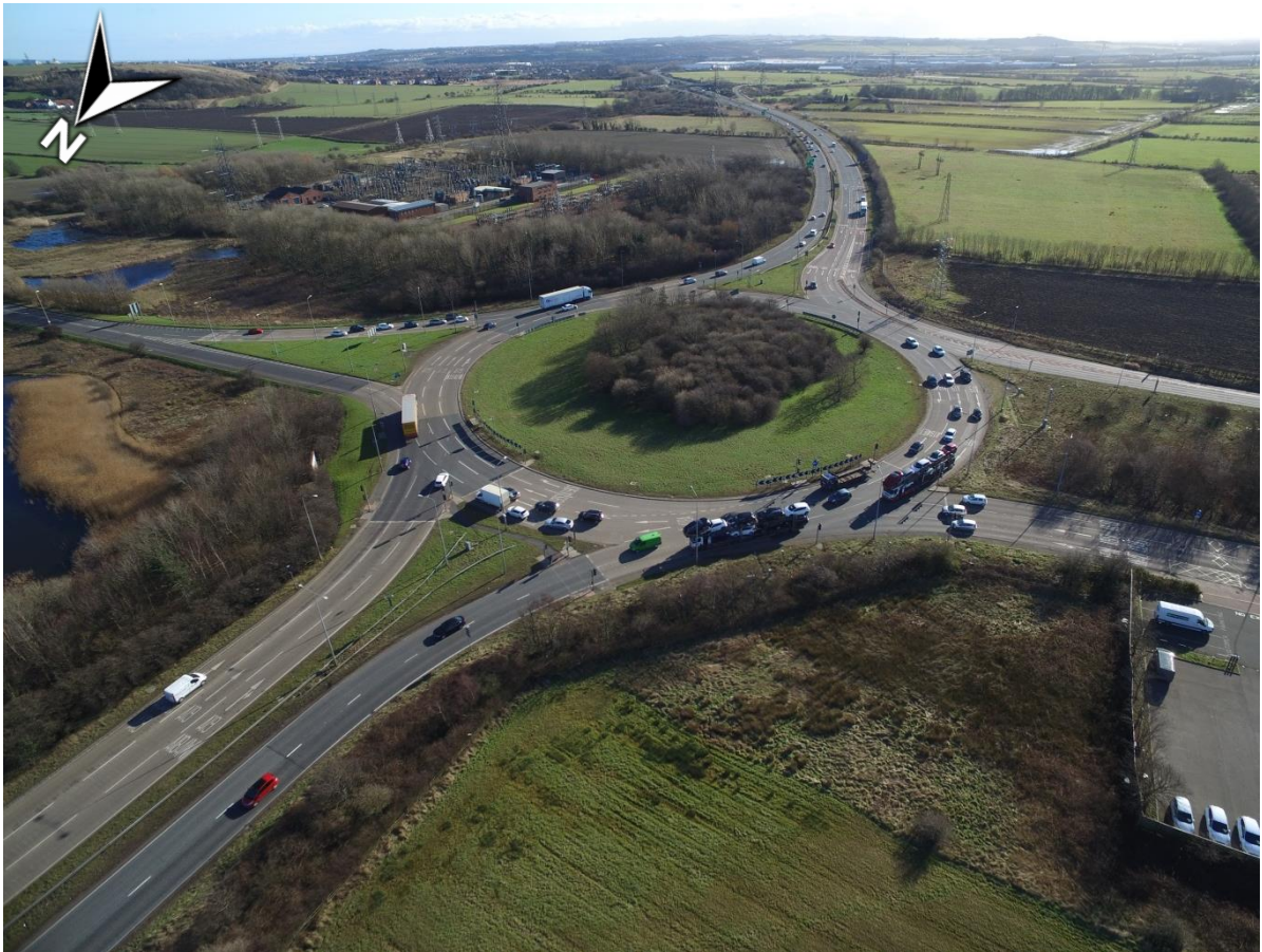
Plate 2-1: Testos junction, looking south towards Downhill Lane Junction
