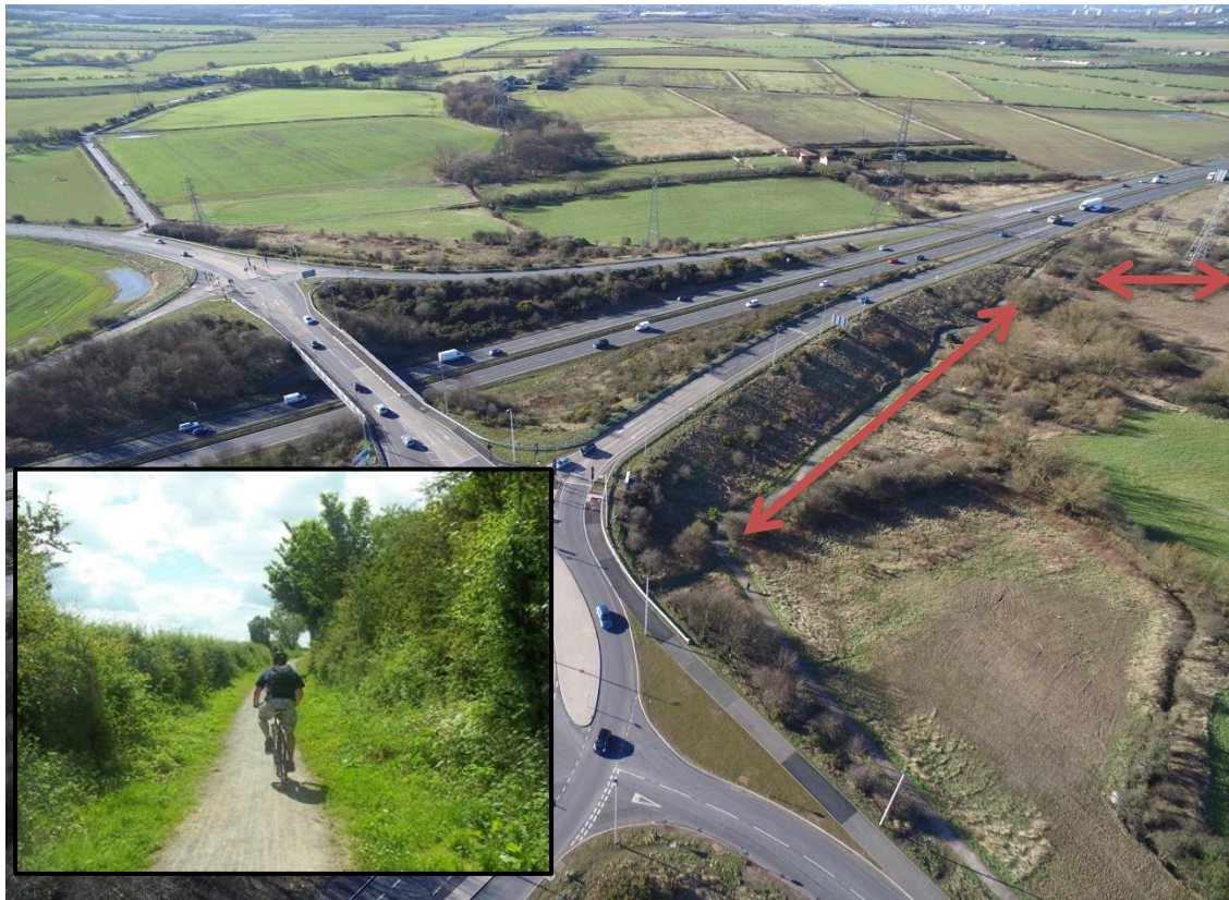
Plate 3-2: Aerial view of Bridleway B46 near Downhill Lane junction. Inset: looking south from near the A184
