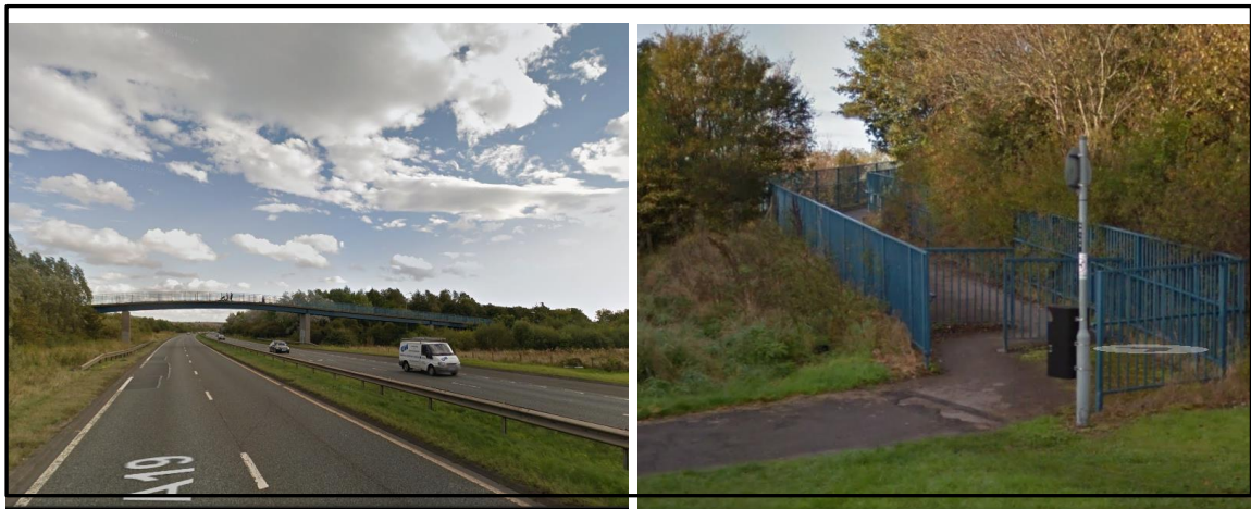
Plate 3-4 Left) Nissan Footbridge from the A19 south-bound Right) Entrance to Nissan Footbridge from Washington Road
